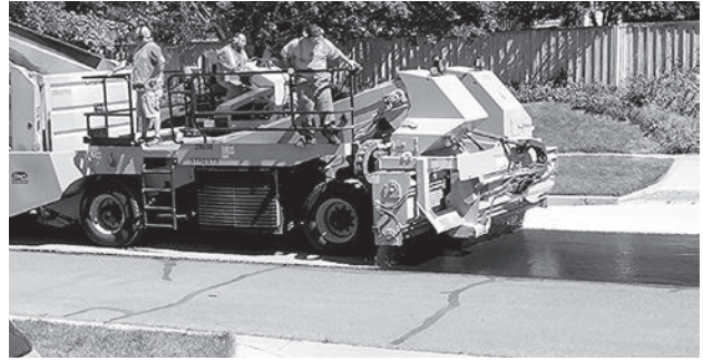
Chip spreader lays down rock chips atop hot asphalt emulsion.
